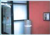
Access Control System
